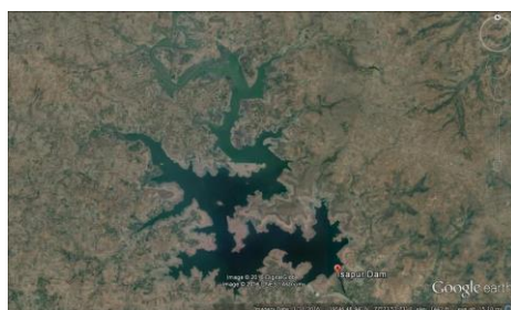
Fig. 1: Google image of Isapur dam
